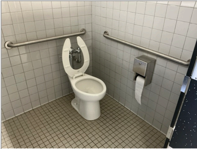
TOILET STALL OVERVIEW
